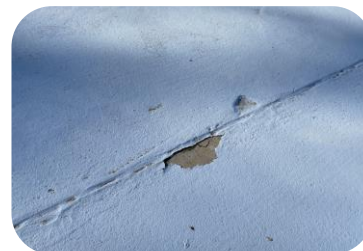
Areas of bare concrete were observed where the pool paint has delaminated.
