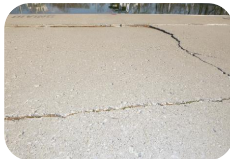
Several areas of the pool deck are in poor condition and need to be replaced.
