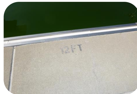
Dive pool depth markers need to be repainted or replaced with tile markers.
