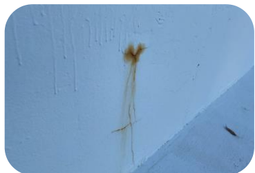
Corrosion exists on the side walls of the recreation pool where it appears the chlorinated water has penetrated the concrete shell and reached the embedded rebar.
