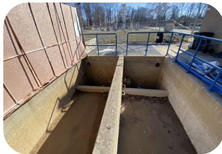
The pools' filtration is an open-air gravity sand filtration should be replaced with either high-rate sand filtration or regenerative media filtration.
