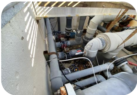
Mechanical system is exposed to the outdoor elements which decreases its expected lifespan.
