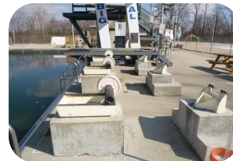
Several of the 1-meter diving boards do not have side rails installed.
