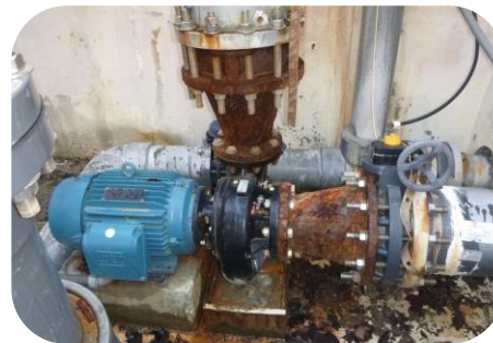
Code requirement for turnover rate which is 6 hours (main pool – 6.15 hours, dive pool – 9.7 hours) is not met with either pool.
