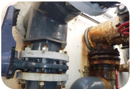
Significant corrosion on piping connections and pipe supports, and the waterslides' pump and strainer basket show similar signs of corrosion.
