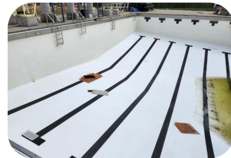
A pool liner/membrane was installed in both pools in 2012 due to significant water loss that was occurring in the main pool which is typically due to failures in the pool structure and/or the original cast iron piping.
