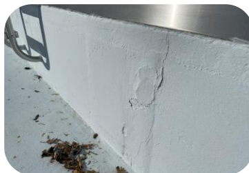
Gaps exist beneath the pool's stainless-steel gutters where it connects to the concrete wall.
