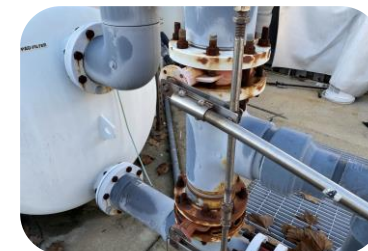
Corrosion exists on components of the recirculation system including the pipe connections, pipe supports, pool pumps and motors, and on the high-rate sand filters.
