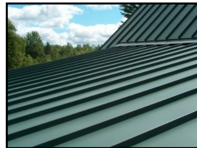
GREEN STANDING SEAM METAL ROOF
