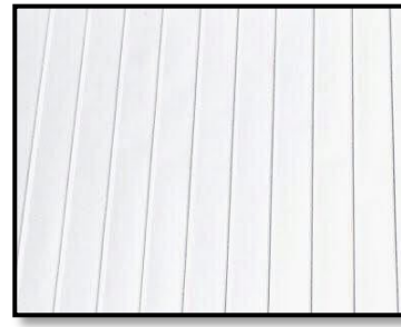
Galvalume Standing Seam Metal Roof
