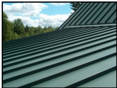
GREEN STANDING SEAM METAL ROOF
