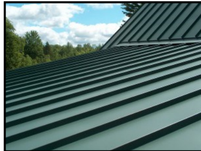
Green Standing Seam Metal Roof
