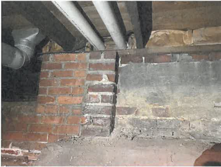
Photo 3: Utilities have open air gaps to the outside.
