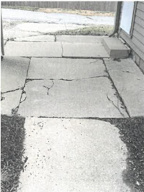
Photo 21: Settlement and cracking of the exterior concrete – between house and detached garage.
