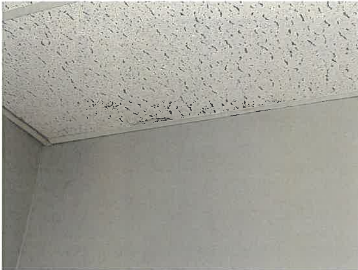
Photo 20: Water marks in the ceiling indicate the roof is leaking.
