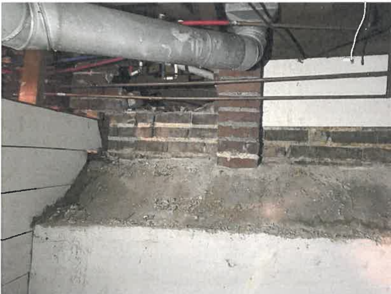
Photo 4: Distressed foundation wall in basement.
