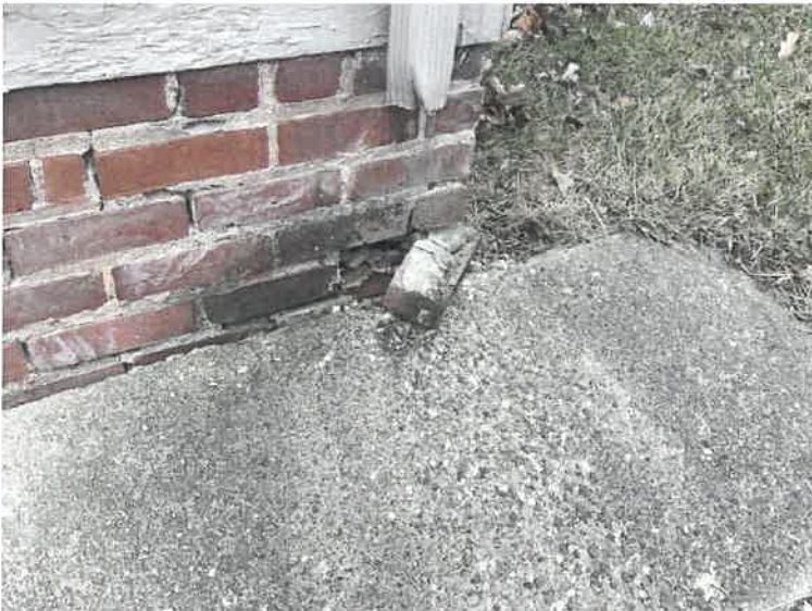
Photo 12: East foundation wall severely damaged, with mortar joints missing.
