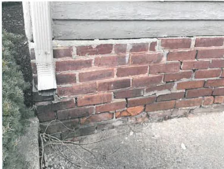
Photo 9: East foundation wall severely damaged, with mortar joints missing.
