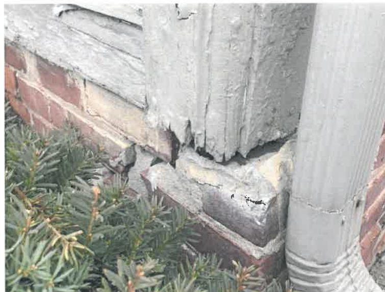
Photo 10: The foundation wall to wood framed wall interface severely damaged at SE building corner.
