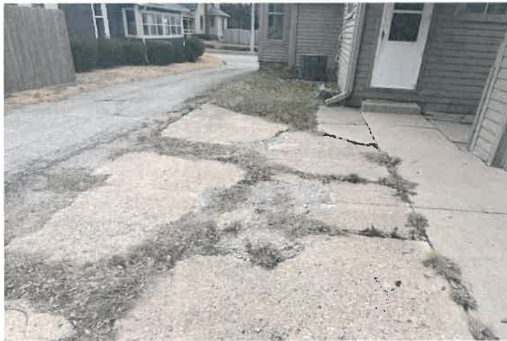
Photo 22: Concrete drive lane distressed at garage entrance.
