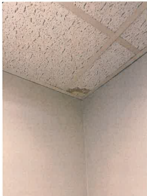
Photo 19: Water marks in the ceiling indicate the roof is leaking.
