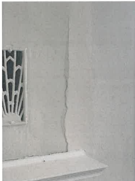
Photo 16: Cracking was observed throughout the interior wall, particularly the south wall. Indicates foundation settlement.
