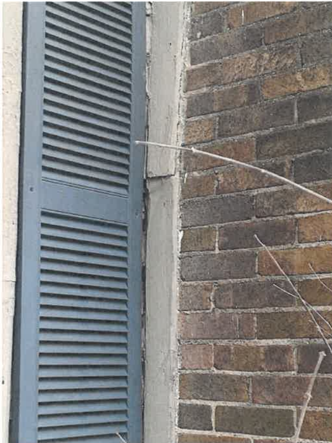
Photo 14: Another view of the chimney pulling away from the main structure.
