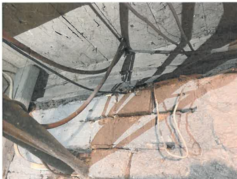
Photo 6: Sill Plate for exterior wall is rotten.
