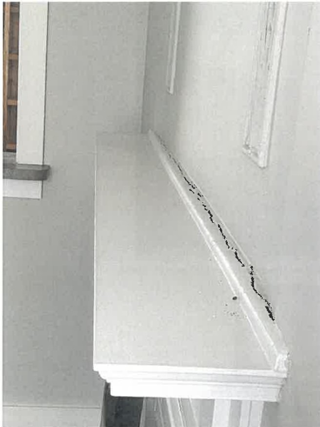
Photo 17: View of wall at fireplace mantle, cracking indicates the chimney is pulling away from the main structure.
