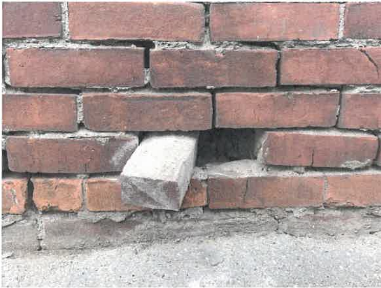
Photo 11: East foundation wall severely damaged, with mortar joints missing.
