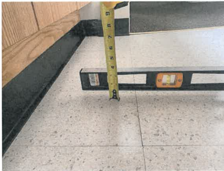
Photo 15: Portions of the interior floor have significant movement/sag.
