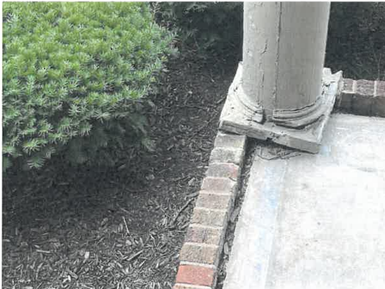
Photo 8: Due to settlement of porch, the column supporting the porch is damaged.
