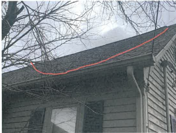
Photo 18: Roof is sagging throughout, the above view is the north side of the building.
