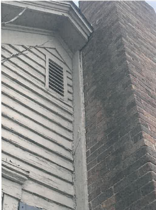
Photo 13: The chimney is settling and pulling away from the main structure.
