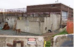
New Grit Removal Tanks
