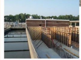
New Wet-Weather Equalization Basin (to be Converted to Primary Clarifier in Phase 2)
