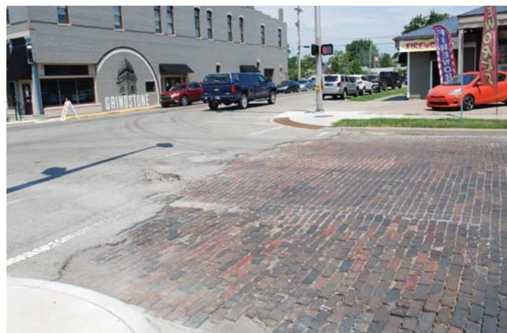
*Example of why a flush concrete band is needed between asphalt and pavers.*
