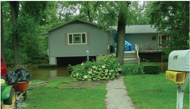
Elevated house during July 2003 flooding.
